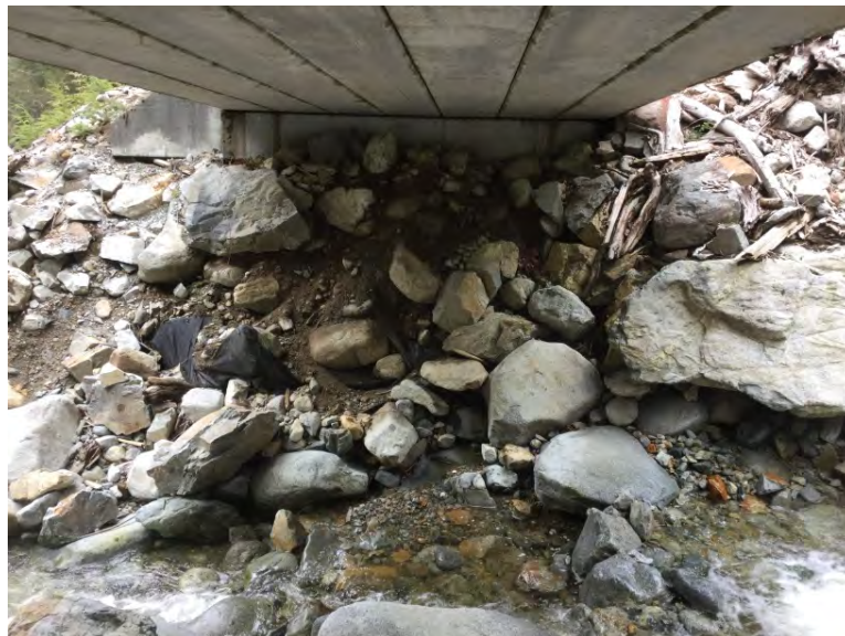
Right Bank Abutment when facing downstream
