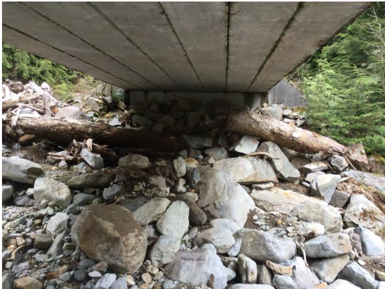
Left Bank Abutment when facing downstream
