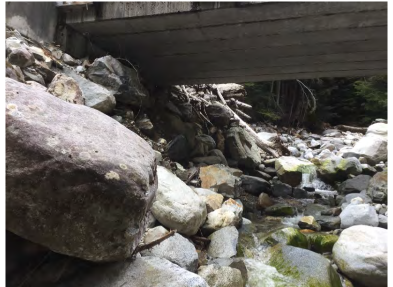
Right Bank Abutment when facing downstream
